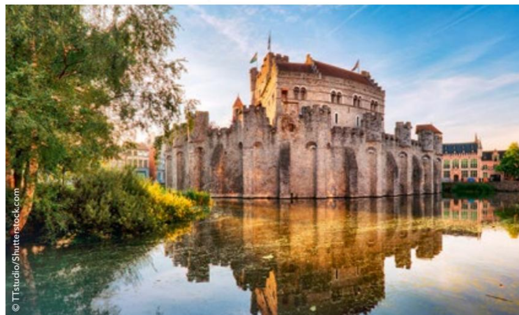
One of the largest water castles in Europe: Gravensteen Castle in the historic center of Ghent
