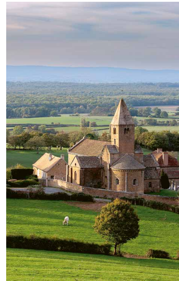
SAINT PIERRE CHURCH, BRANCION
